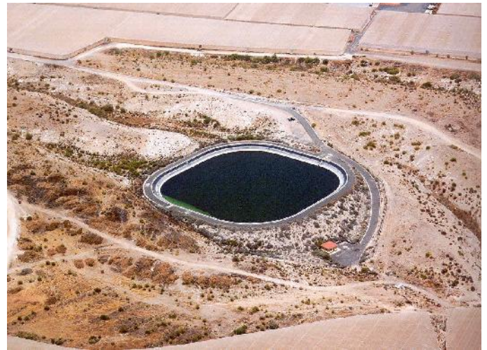
Figure 2. Reservoir of “San Isidro” waterproofed with HDPE.
