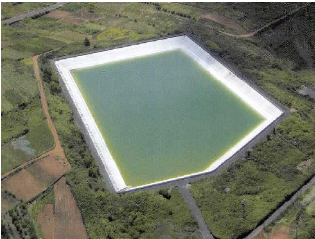
Figure 1. Reservoir of “Los Llanos de Mesa” waterproofed with PVC-P.
