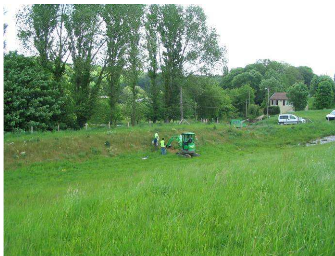
Figure 2. Dam to prevent flooding.
