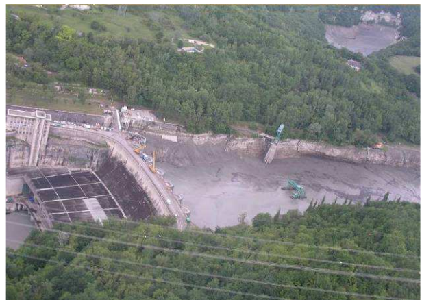
Figure 8. Genissiat dam during flushing – bottom gate on the right bank, photo CNR
