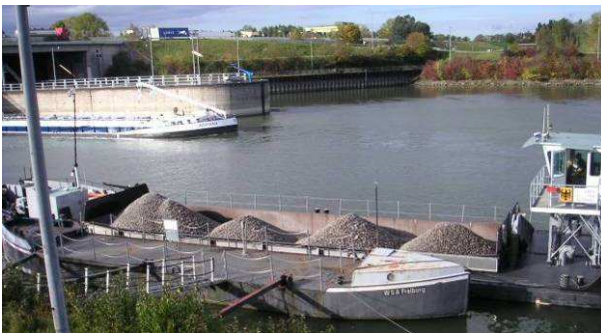
Figure 10. Nourishment of the Rhine River by barges of gravel, photo L. Schmitt
