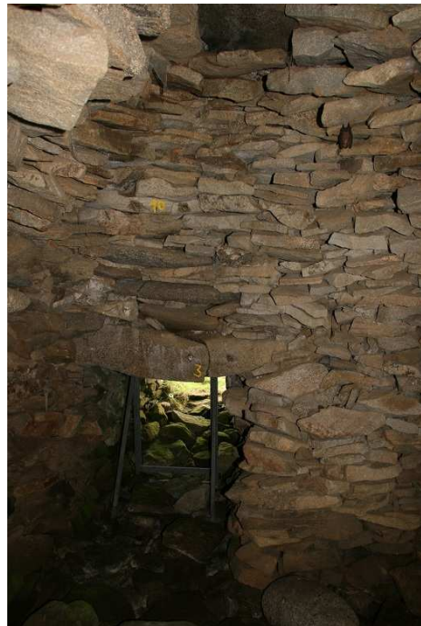
Figure 3: Inside view of the central chamber
