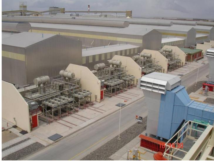
**Figure 4. Example of an Alstom Grid AC/DC conversion substation (Aluar, Argentina)**
