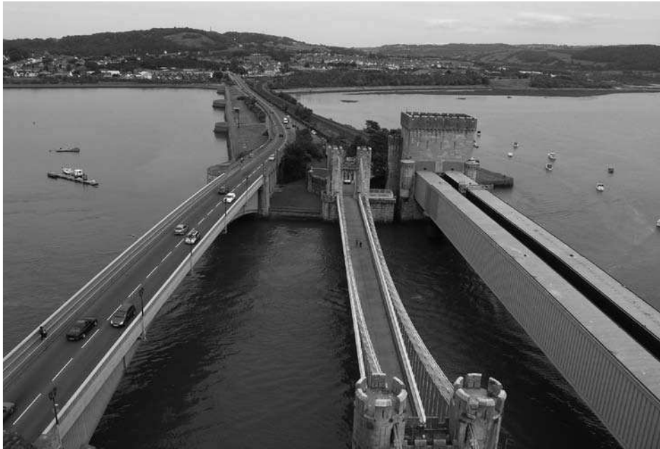
Conwy Bridge, North Wales.
