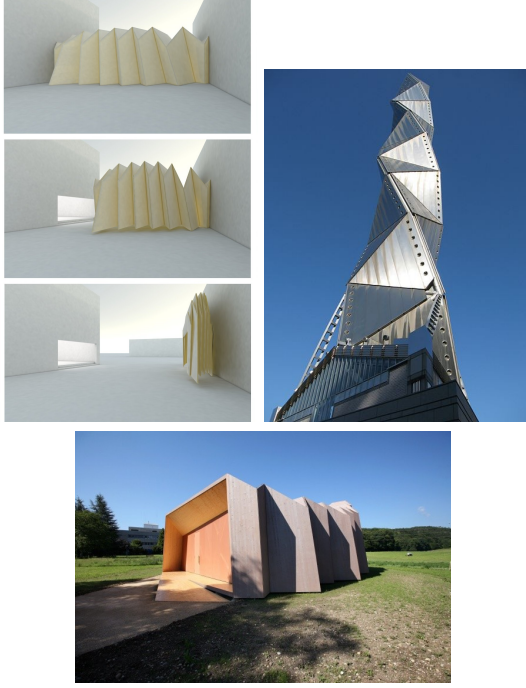
Figure 1: Using folds in architecture. Top left: kinematic aspect of a foldable gallery (T. Tachi [26]); top right: morphogenetic aspect of the Art Tower Mito (A. Isozaki, image by Korall, Creative Commons 2006); bottom: static aspect for the Saint Loup Chaptel (Localarchitecture / H. Buri, Y. Weinand / D. Mondada, 2008 [1])
