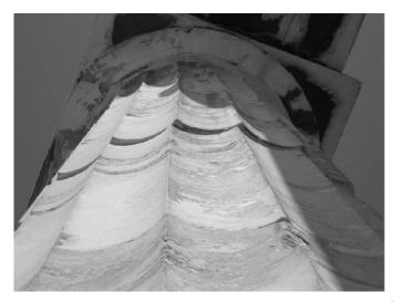
Figure 12. Mechanical damage of a column of Parthenon (see also Bouras et al. [24]). The relative displacements and rotations of the column drums corroborate the wobbling motion and the three dimensional dynamic response of these articulated systems.
