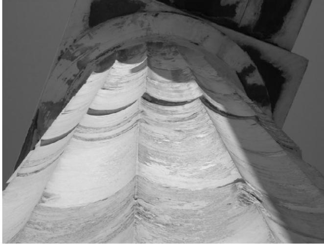
*Figure 12. Mechanical damage of a column of Parthenon (see also Bouras et al. [24]). The relative displacements and rotations of the column drums corroborate the wobbling motion and the three dimensional dynamic response of these articulated systems.*
