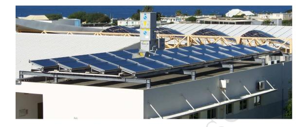
Fig. 4 : Solar collector field of the solar cooling process
