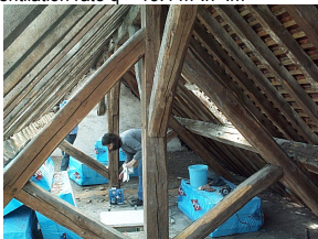
Figure 2. Roof trussing before renovation (total wood surface 84 m 2 , volume 65 m 3 ).
