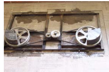
Fig. 8 Photography of the Installation of the Exciter
