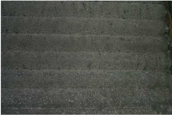
a) Heavily fouled finned tube bank
