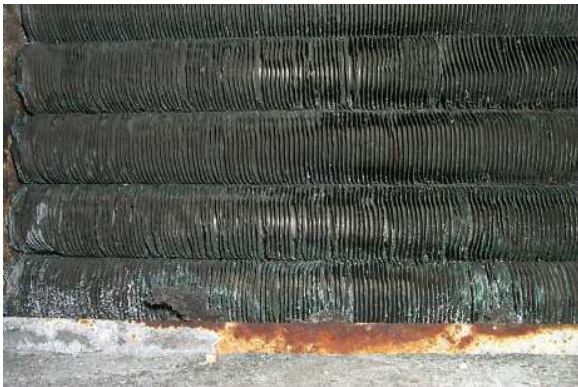
b) Finned tube bank after cleaning
