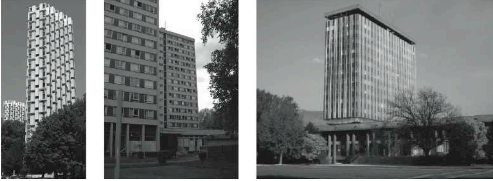
Figure 3: General view of the Mont-Blanc Tower (MBT, left), the ARPEJ Tower (AT, centre) and the Grenoble City Hall building (CHB, right).
