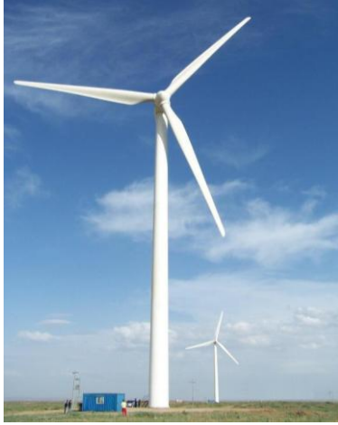
Fig. 5. 1.5-MW wind turbine illustration.
