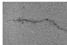
Figure 1: Initial image example ( I(x, y, 1) ) – The crack corresponds to a local low-contrasted heterogeneity.
