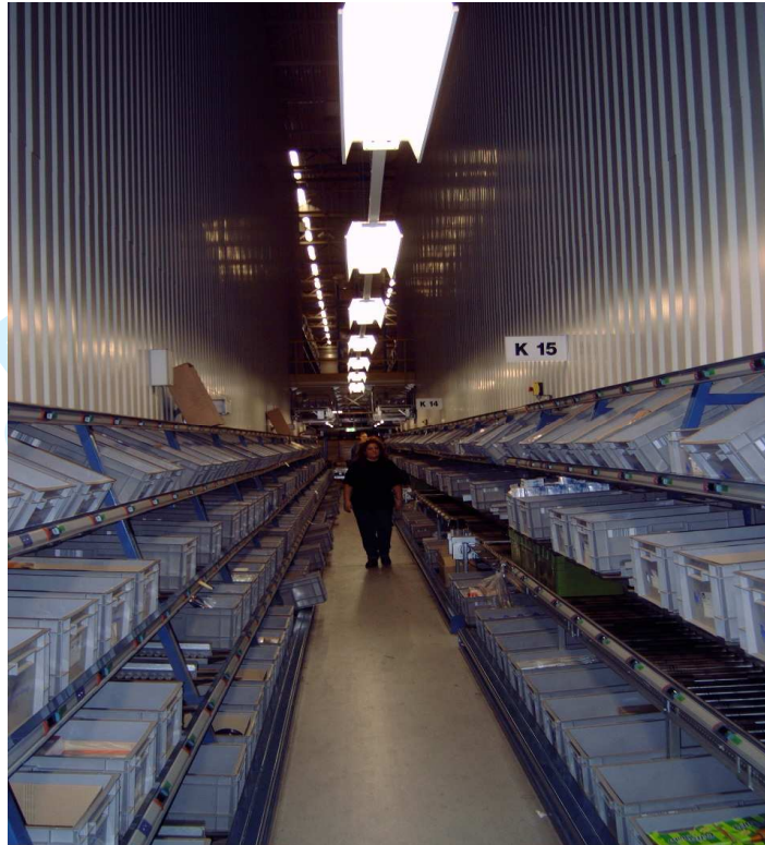
Figure 1: An illustration of a DSS at Nedac Sorbo : the S/R machines replenish the pick bins from a bulk storage area behind the walls.
