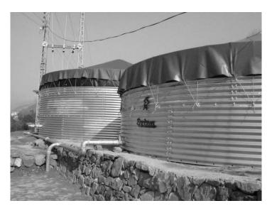
Figure 3: Emergency batch sedimentation tanks used in Gahri Dupatta.
