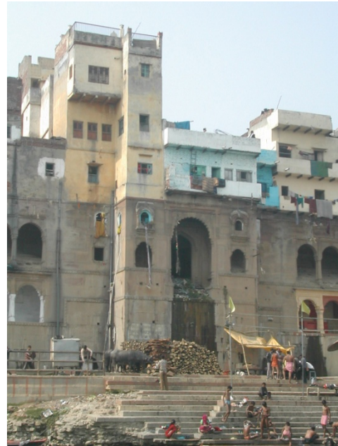
Figure 7: Overflow of sewage causing destruction of palatial houses
