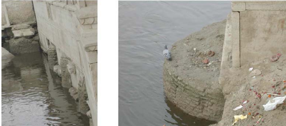
Figure 3: Masonry wells as foundation piles in Vrindavan
