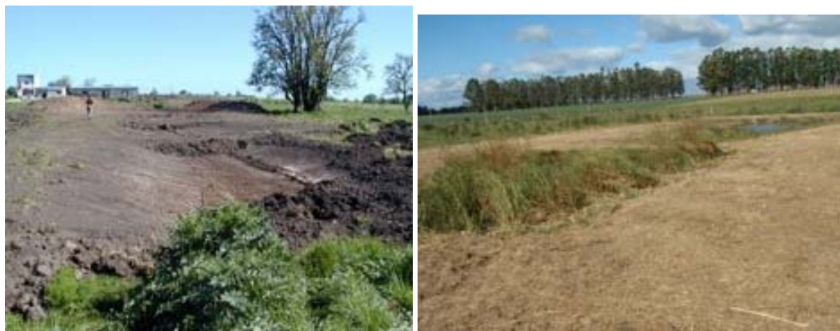
Figure 6: Images of the construction of the wetland and the vegetated areas.
