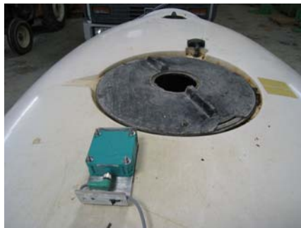
Figure 4: Tank level sensor © Cemagref 2009
