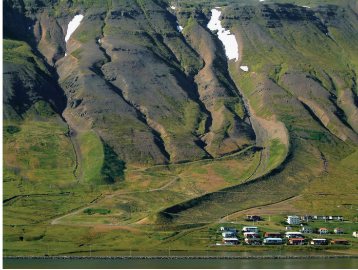
Figure C2: Deflecting dams at Siglufjörður, northern Iceland. The larger Strengsgil dam is 18 m high and the smaller Jörundarskál dam is 15 m high. (Photo: Reynir Vilhjálmsson.)
