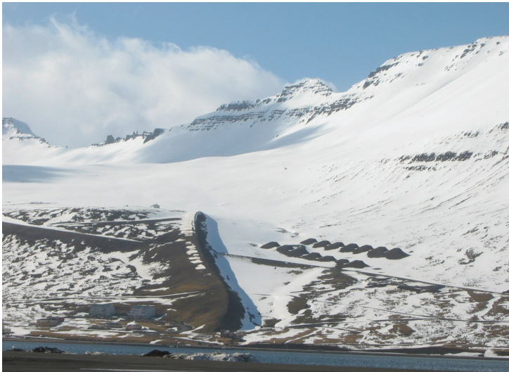
Figure 15.1: Deflecting dam and braking mounds at Seljalandsmúli in Ísafjörður, northwestern Iceland. The dam is 650 m long and 16 m high, and the braking mounds are 7 m high. The total volume of fill material in the dam and mounds is 360,000 m 3 . (Photo: Tómas Jóhannesson.)
