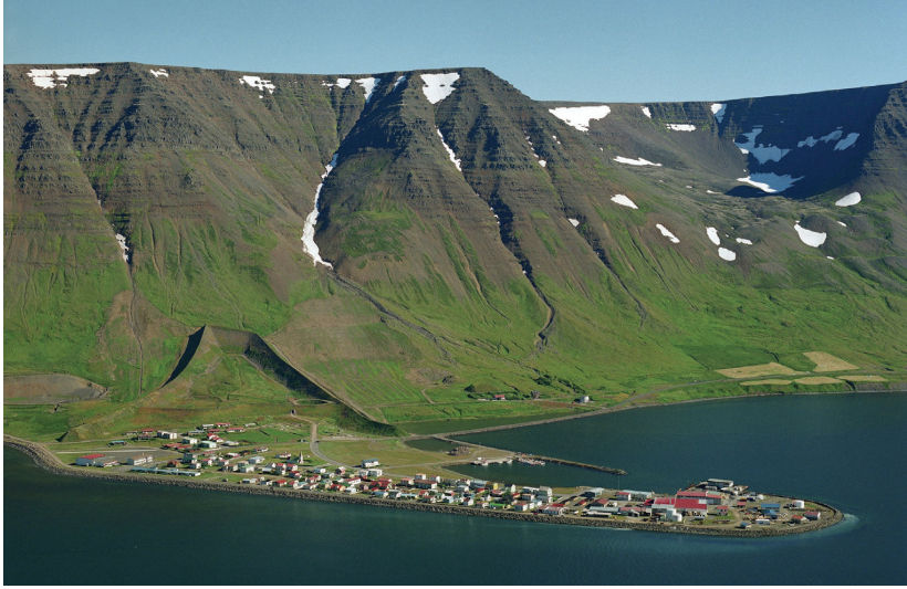
Figure 3.3: Two deflecting dams and a catching dam at Flateyri, northwestern Iceland. The deflecting dams are 15–20 m high and the small catching dam between them is 10 m high. The dams were built after a catastrophic avalanche in 1995 that killed 20 people. (Photo: © Mats Wibe Lund.)
