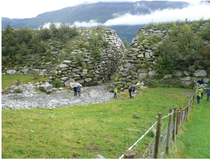
Figure 15.6: A river outlet through a dam (photo: Karstein Lied).
