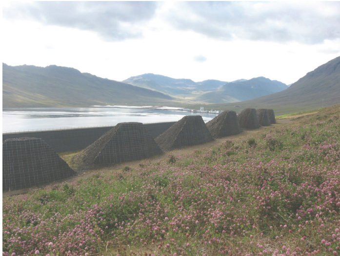
Figure 15.8: A row of 10 m high braking mounds at Neskaupstaður (see map in Fig. 15.7) (photo: Tómas Jóhannesson).
