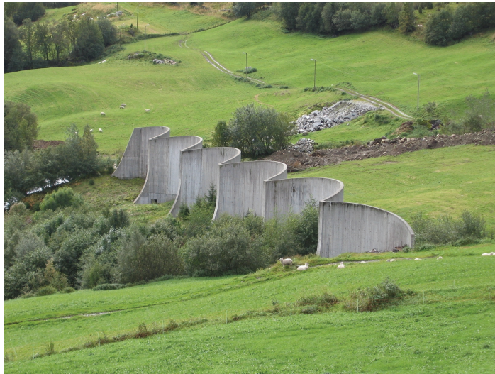
Figure 15.11: A retaining dam made of six 20 m wide and 10 m high reinforced concrete shells at Ullensvang, Norway (designed by NGI and Instanes AS, Norway). Maximum design avalanche impact force is 92 kPa. Each shell has four vertical steel anchors, each with a capacity of 2800 kN, drilled 12–14 m into the bedrock. Tilting moment on each shell is 59,000 kNm, and shear force is 8500 kN. (Photo: Ulrik Domaas.)
