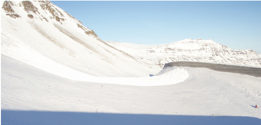
Figure 3.2: A catching dam at Brún in Bjólfur in Seyðisfjörður, eastern Iceland. An avalanche that fell on 9 February 2008 and stopped just at the dam face can be seen. The dam is 20 m high with a 10 m high very steep upper part. (Photo: Emil Tómasson.)
