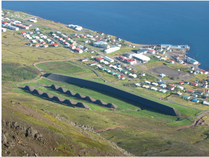
Figure D2: The braking mounds at Neskaupstaður and the catching dam behind them. Each mound is 10 m high and the catching dam is 17 m high. (Photo: Tómas Jóhannesson.)
