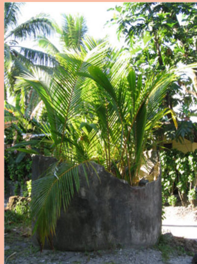
Box Fig. 1.5a.4 Broken tank: Rainwater catchment tanks are prone to cracking and breaking when not maintained and kept full of water. A broken tank on Funafuti Atoll collects organic material and makes a fertile home for new palm growth (Photo credit: Heather Lazrus)
