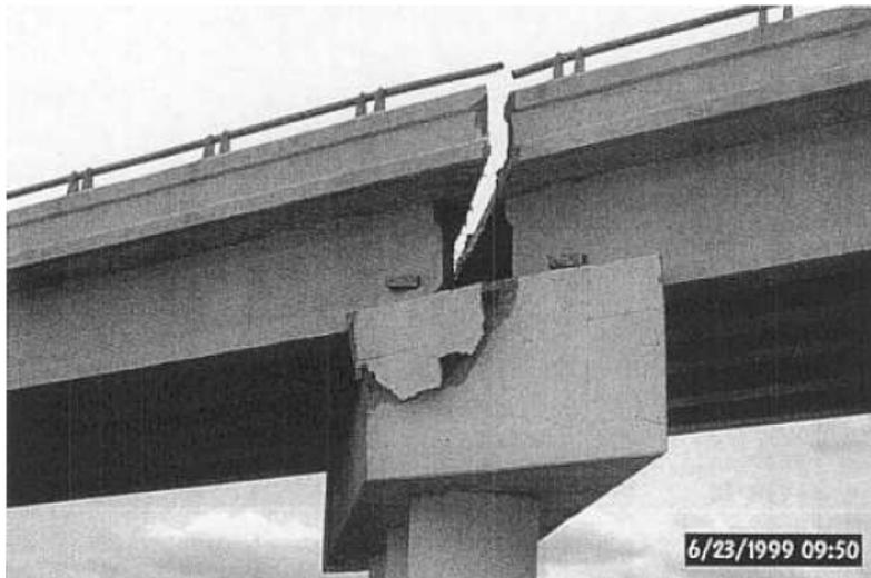
Figure 1. Damage of a skew bridge after the Tehuacan 1999 Mexico earthquake [6].
