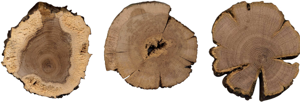
Fig. 4. Examples for different types of distribution and dissemination of decay in round posts. Left: Decay starting from the sapwood. Centre: Decay starting from the central heartwood. Right: Decay starting mainly from radial cracks.
