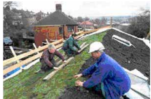
Fig (3). In the Hockerton Project (UK, 1996) roofs were covered with soil rather than tiles to increase energy efficiency by trapping heat. The soil acts as a giant radiator.
