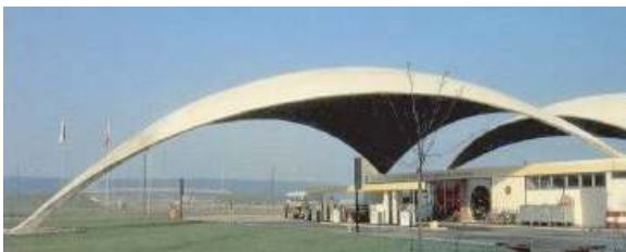
Figure 8-a. Gazoline station, Deitingen, Switzerland, 1968.
