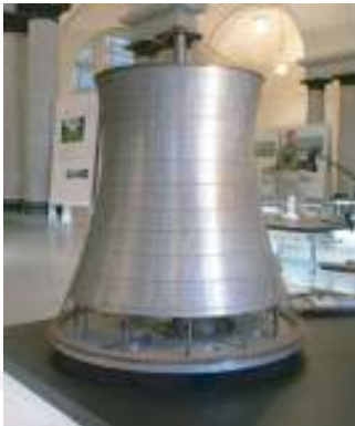
Figure 6. Cable net dry cooling tower, Schlaich Bergemann & Partners, 1974.
