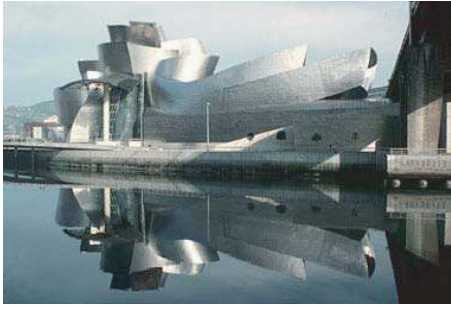
Figure 14-a. Guggenheim Museum, Bilbao, Spain, 1997.
