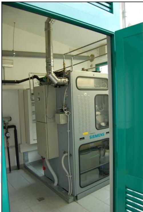
Figure 1. Installation of the 5kW Siemens Generator in Turbocare Spa.
