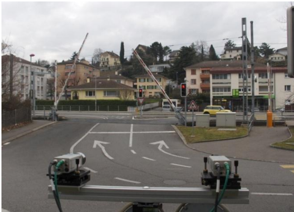
Figure 6. A level crossing (in Ecublens-Switzerland): obstacle detection system that utilizes stereo cameras and image processing technology.
