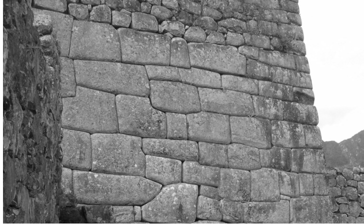
Figure 2. Interlocking blocks at masonry wall in Peru (I.Vardoulakis 2006).
