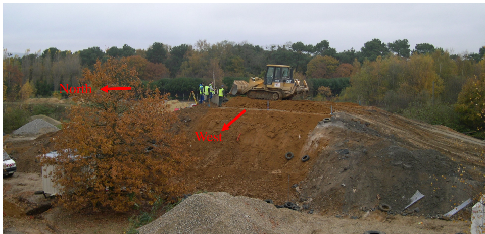
Figure 1. Rouen test embankment near completion.
