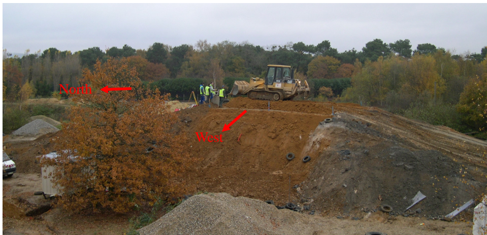
Figure 1. Rouen test embankment near completion.
