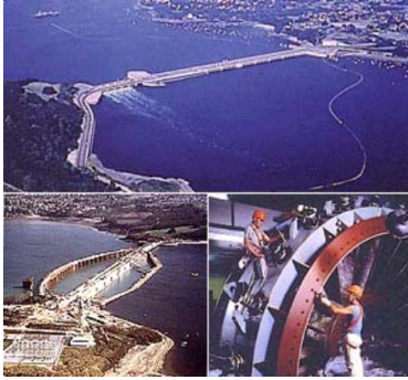
Fig. 2. La Rance tidal power station [6].
