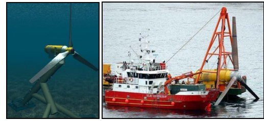
(a) E-tide turbine. (b) Installation. Fig. 9. The Blue or E-Tide concept [© Strøm AS].
