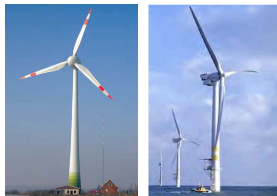
Fig. 2. Currently largest onshore wind turbine and offshore installations [6].
