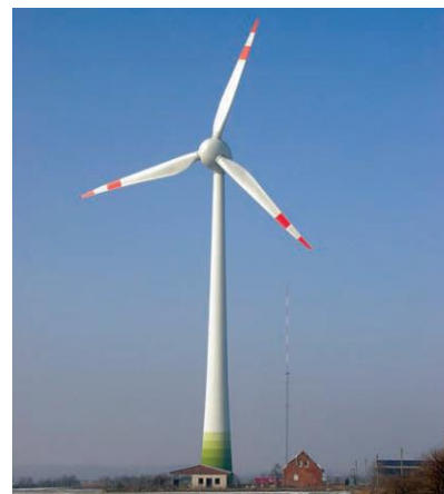
Fig. 13. Largest wind turbine (currently): Enercon E-112 with a rotor diameter of 112 m and a nominal power of 4.5 MW.
