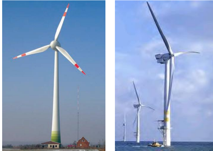
Fig. 2. Currently largest onshore wind turbine and offshore installations [7].
