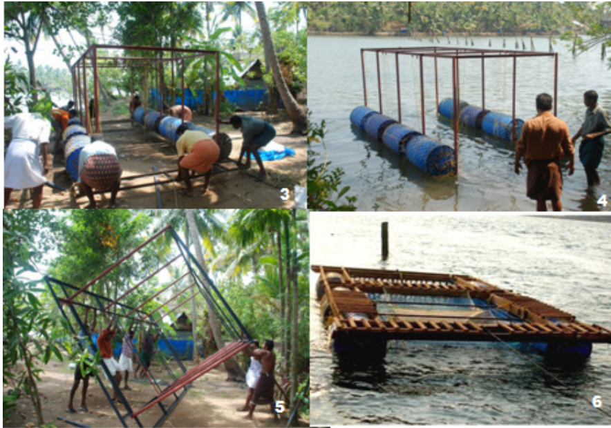
Fig 3-5: Fabrication of the “Microsate” cage by the fisherfolks
