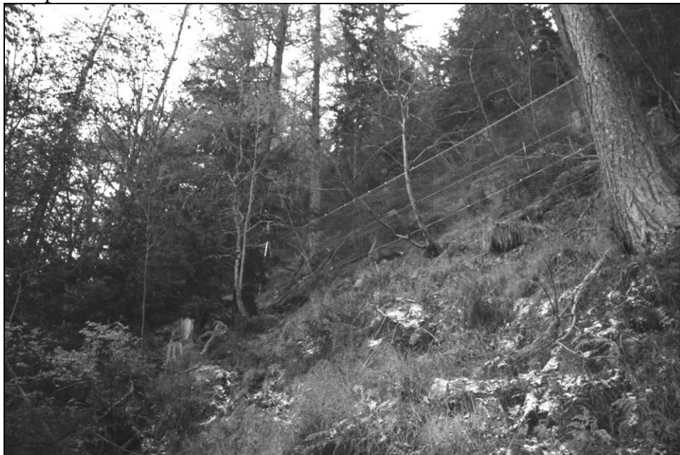
Fig. 7. Fence installed in a pilot forest. Chamonix, France (2009)
