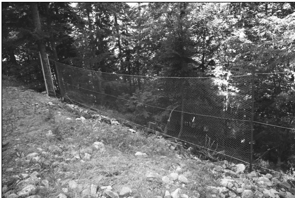
Fig. 1. Fence installed for real size experiments in Vaujany, France (2008)
