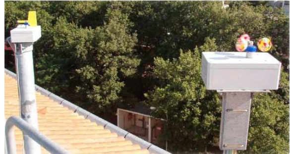
Fig 12: Anemometer and waethercock sensors on the roof of the University.
