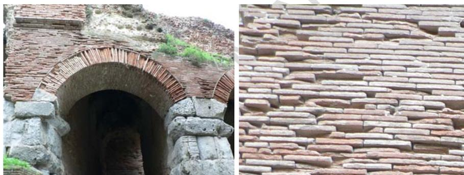
Figure 4: An example of Roman masonry (Anfiteatro Flavio, built in the second half of the first century A.D. under Emperor Vespasiano at Pozzuoli, Naples. Photo by D. Bigoni). A detail is shown at right of the masonry in the upper left part of the figure at left.
