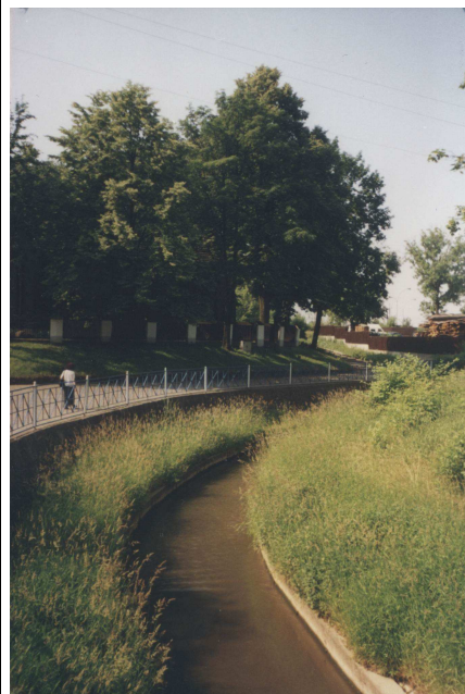
d) improved artificial river cross-section, with low flows channel and bank armoring with Kostecki elements (built in 2003 ; river Wątok in Tarnów, Poland) : riverscape type II
