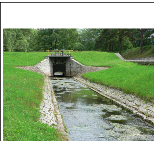
a) upstream view of Krzeszow embankment dam (Poland, height 3.3 m) – lateral spillway on the right
