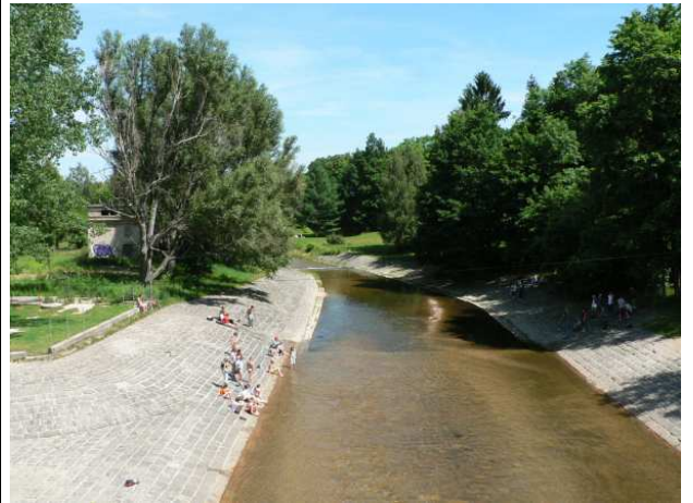
b) armoured stretch of river downstream early XXth century dry dam (Norwegian Park, Jelenia Góra, PL) : type I
