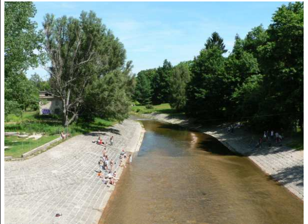
b) armoured stretch of river downstream early XXth century dry dam (Norwegian Park, Jelenia Góra, PL) : type I
