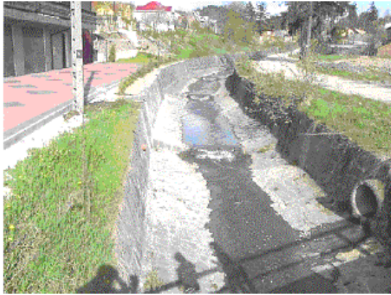
a) stonework : U-shaped early XXth century channel (river Słonka in Rabka, PL) : type I
