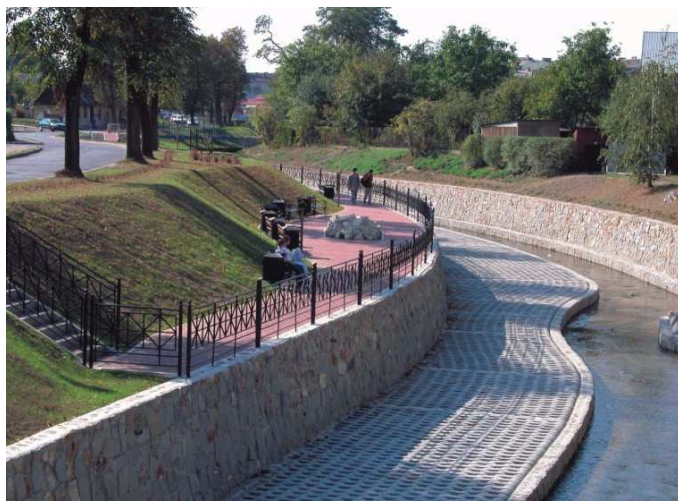
a) stonework : U-shaped early XXth century channel (river Słonka in Rabka, PL) : type I
