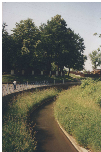
d) improved artificial river cross-section, with low flows channel and bank armouing with Kostecki elements (built in 2003 ; river Wątok in Tarnów, Poland) : riverscape type II
