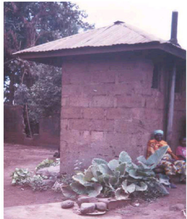
High standing latrines (VIP)
