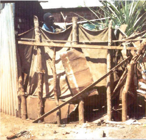
Unroofed flimsy latrines ("passport size")
