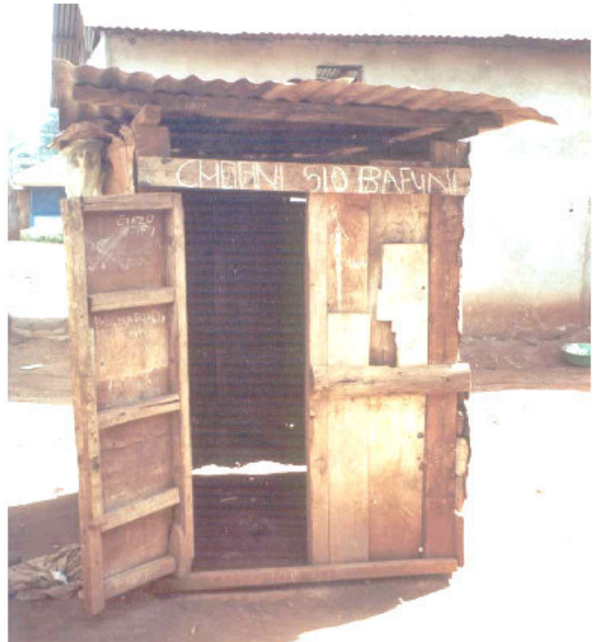
Low standing latrines
