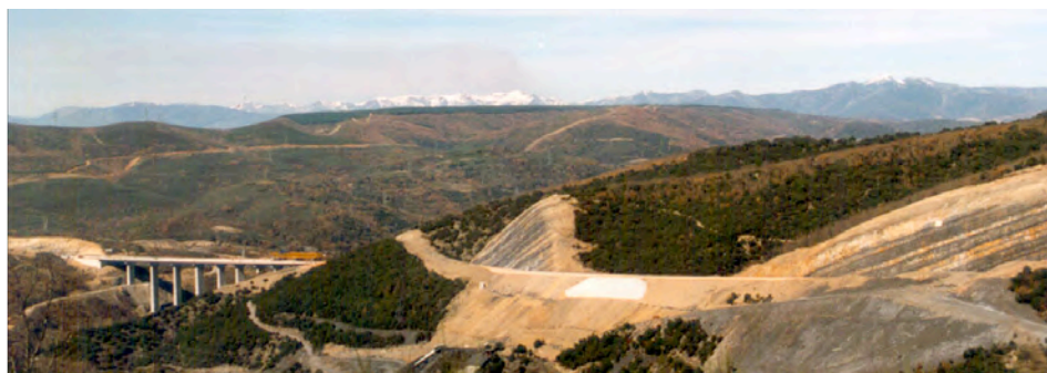
Figure 39. Bad integration of a transport infrastructure in the landscape or natural environment
