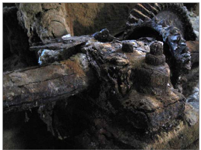
Figure 21: Photograph of bearing and distorted axes (2007)
