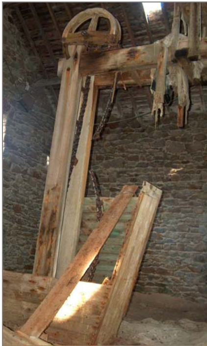
Figure 16: Photograph, Bucket chain (2007)
