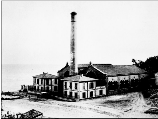
Fig. 11 - The Fontvieille power plant
