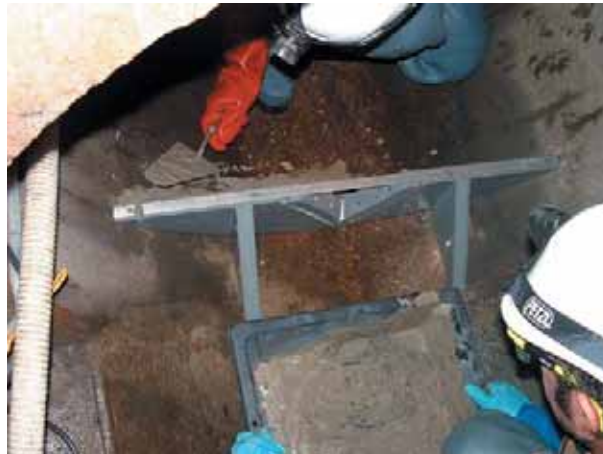
Figure 6 Installation of the V-shaped weir
