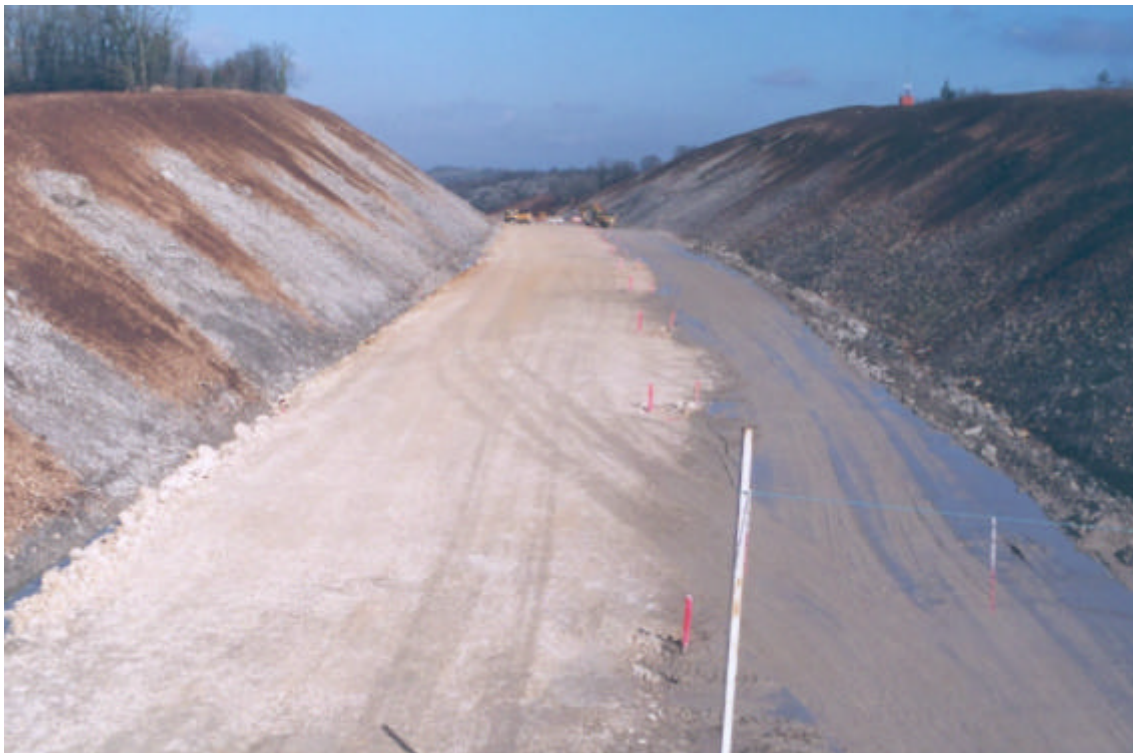
Picture 2 : Newly created embankment before revegetation process. You can see that few quantities of ground was brought back on the top of the embankment while the bottom remained stony.
