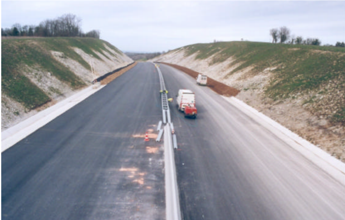
Picture 3 : The same site, one month after sowing in spring. Plantlets appeared on zone covered with ground.
