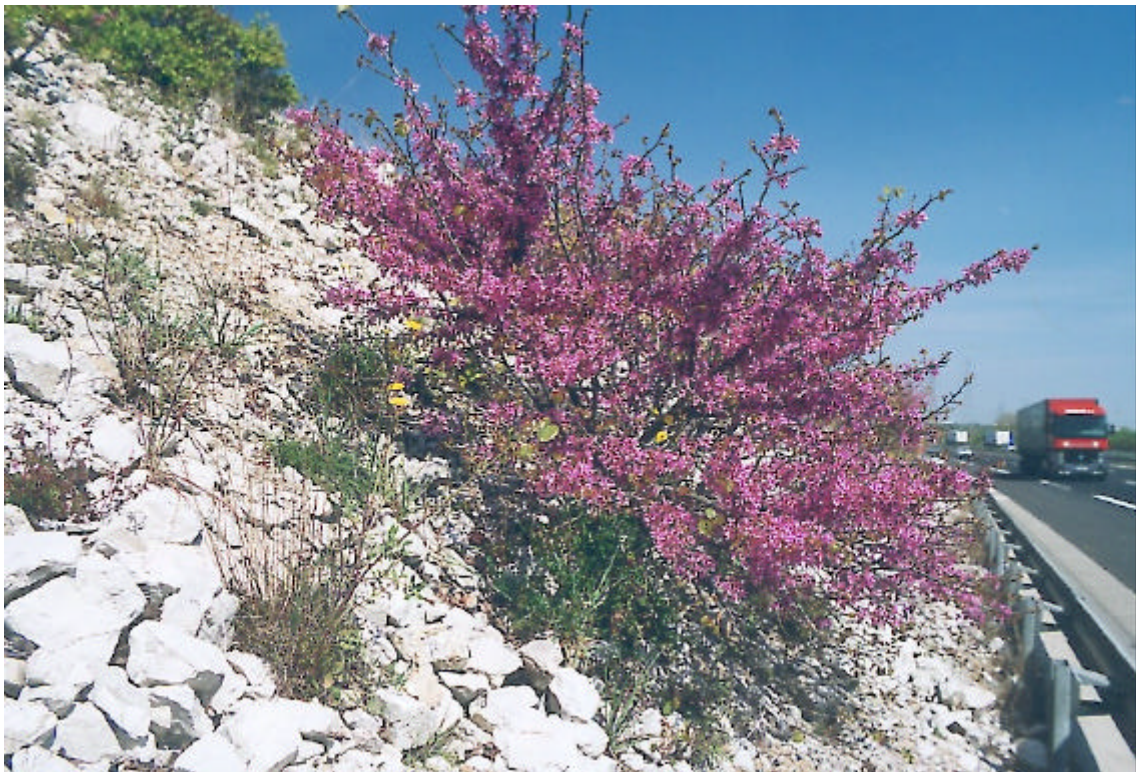
Picture 8 : Cercis siliquastrum , 20 years after sowing along a highway in south of France near Spain. The embankment is not completely covered by vegetation, nevertheless, roots stabilize the soil and the side road is completely integrated into the landscape.
